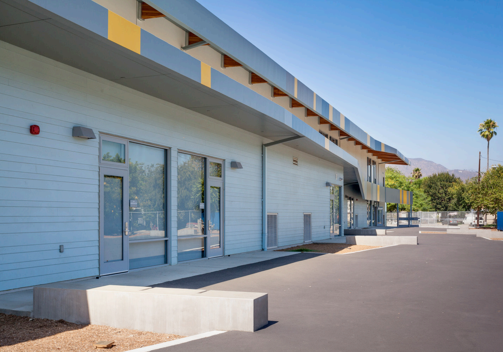
Shade Overhangs On South Side of Building
